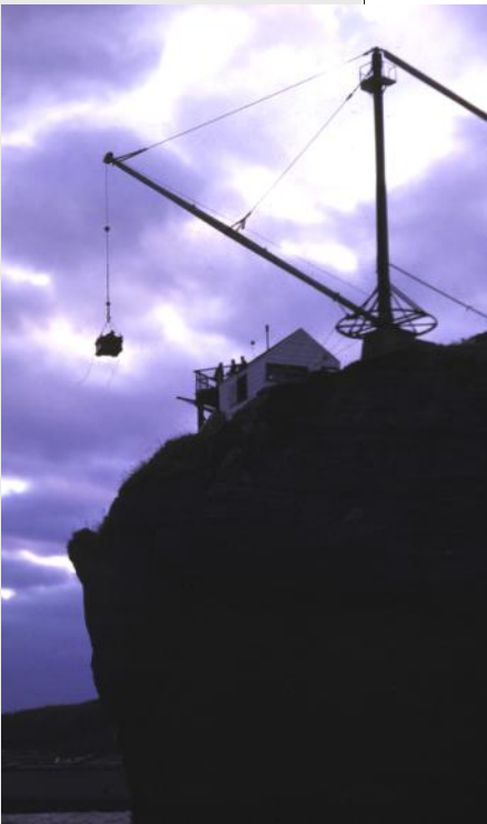
Fig. 2. Cliff top crane transports people and supplies to and from the island.
